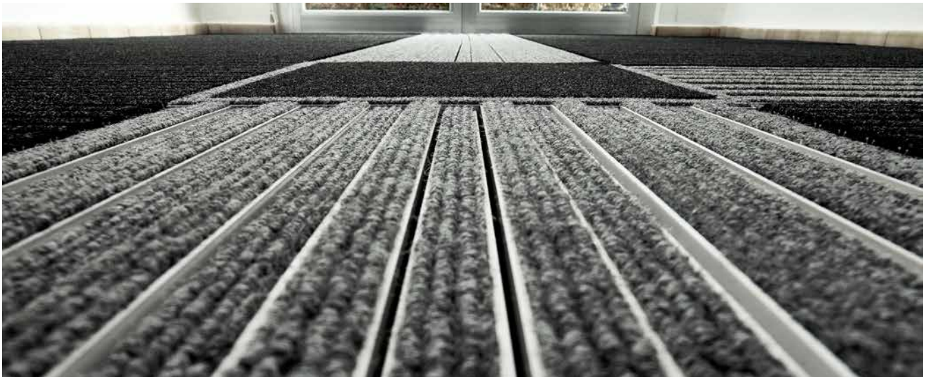
Aluminium profiles with slightly different heights running along the direction of traffic can be felt with the soles of the feet as well as with canes.
